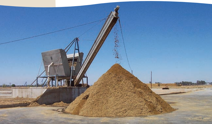
Mechanical screen removes coarse solids from manure flush water.
