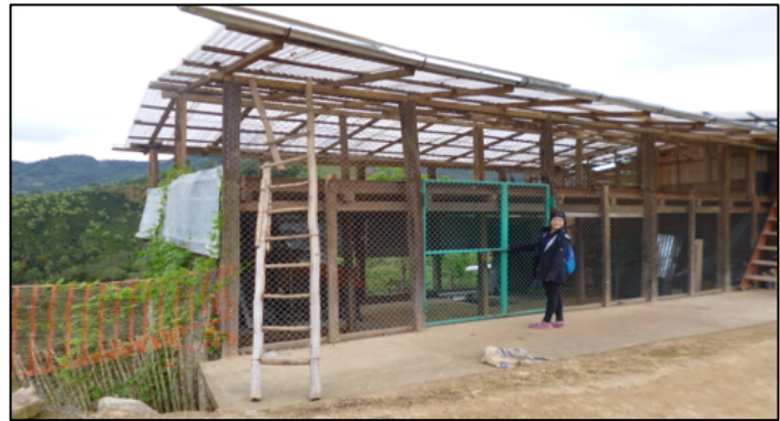
Figure 10: A Calamina Transparente Solar Dryer
