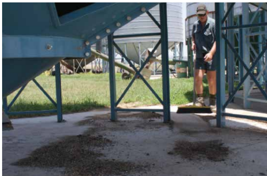
Photo 7: A concrete slab under silo makes cleaning up spilled grain much easier.
