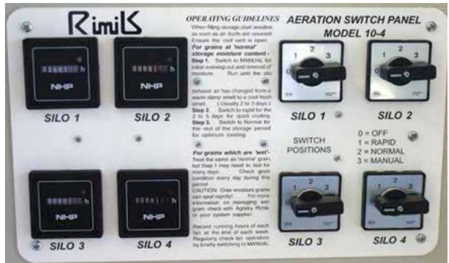
Photo 11: Automatic aeration controllers such as this one are not only the most effective way to cool grain, one unit can manage up to 10 storages.
