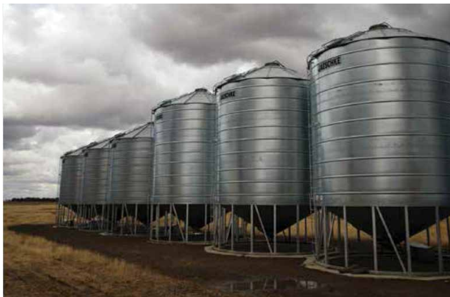
Photo 1: It is important to pressure test all silos used on the farm, even those that are labelled as ‘sealed’.
