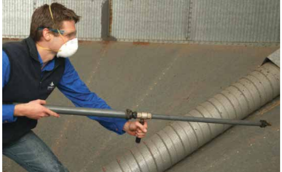
Photo 6: Clean silos, including the silo wall, with air or water to provide a residue-free surface to apply structural treatments.
