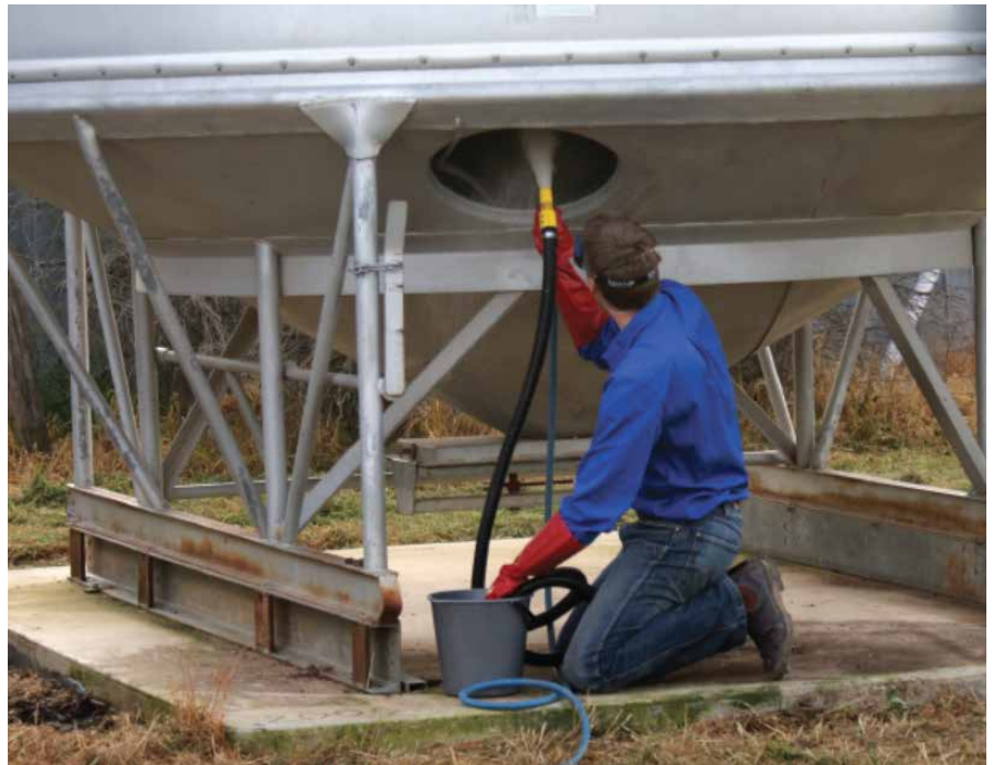
Photo 8: A blow/vac or air venture gun is the best applicator for inert dusts. Aim for an event coat of diatomaceous earth across the roof, walls and base.
