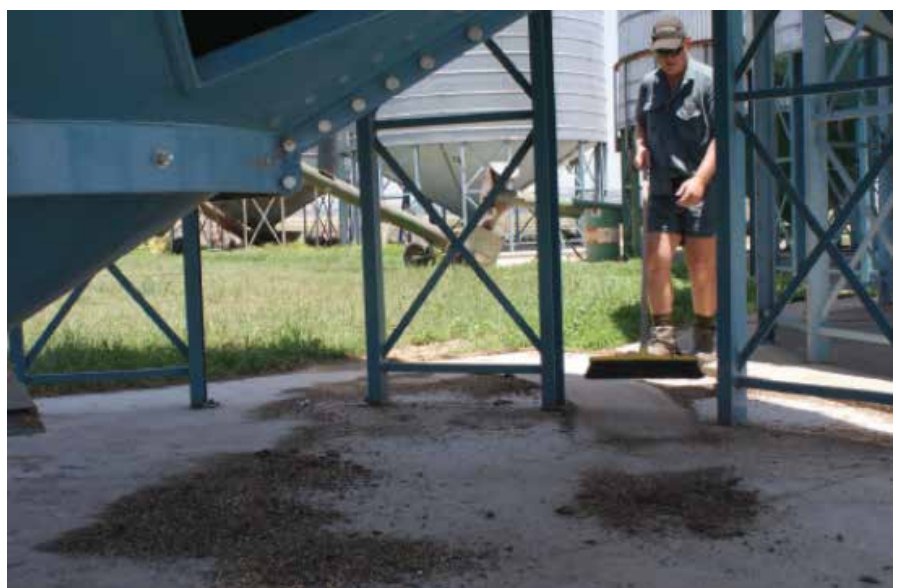
Photo 7: A concrete slab underneath silos makes cleaning up spilled grain much easier.
