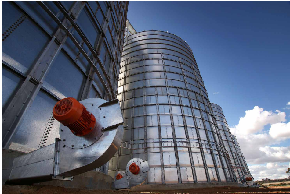
Figure 8: Aeration markedly reduces grain temperature. (Photo: Kondinin Group)
