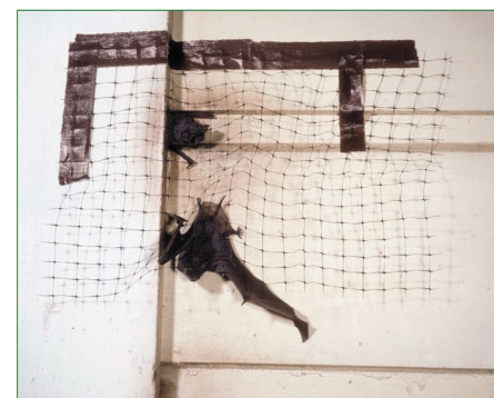
Figure 5. A mesh net is a simple way to exclude bats from a structure.
