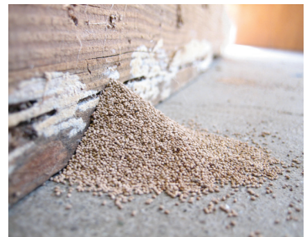
Figure 4. A pile of drywood termite fecal pellets on a horizontal surface. (R.L. Tabuchi, U.C. Berkeley)
